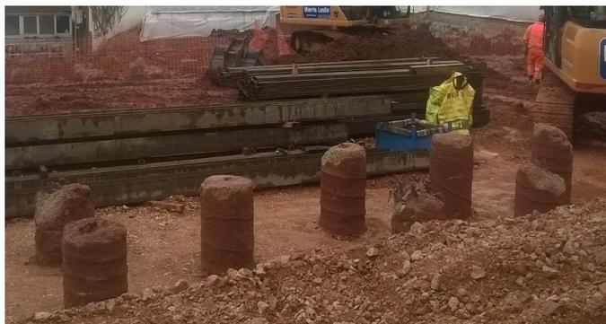
The excavated the piles will be cropped to the required cut off level exposing the reinforcing so that it can be tied in to the pile cap reinforcement.
