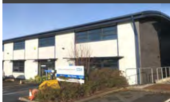
Unit 2 Bay House
