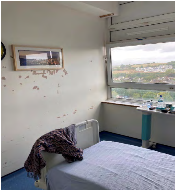
Figure 4-13 - Existing Ward accommodation
